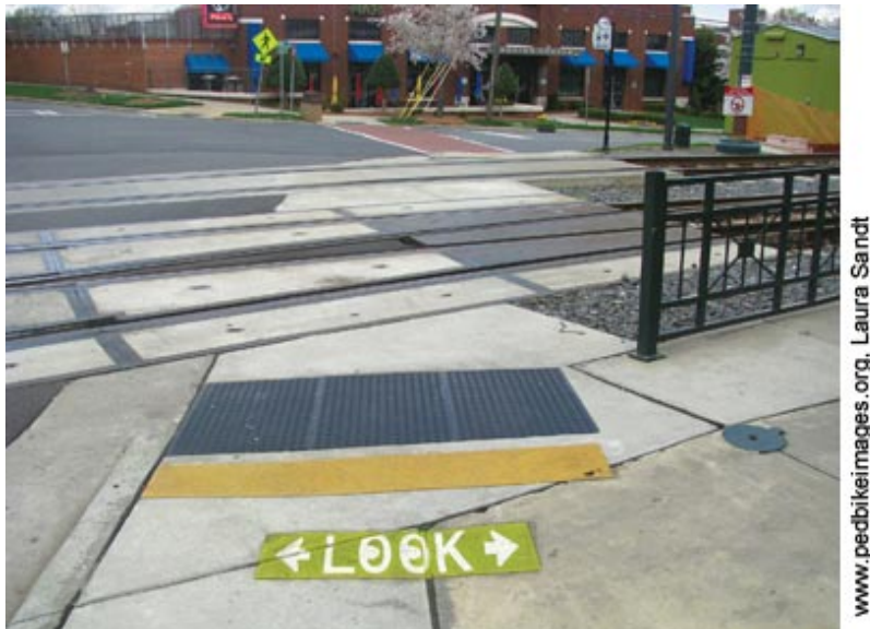
The researchers found that the "Look" pavement stencil, shown here, proved to have low effectiveness in terms of increasing pedestrian safety.
