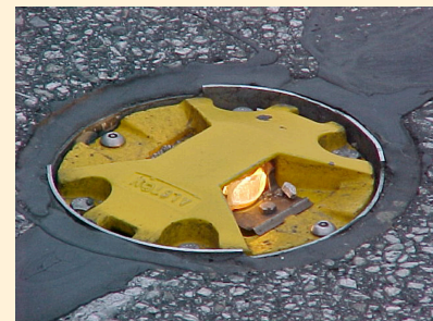
An in-pavement flashing warning light
