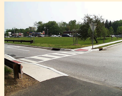
Crosswalk with newly painted striping at the time of the second evaluation
