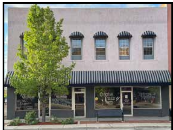
610 - 612 Main Street, Turner House/St. James Hotel. The application of stucco to the exterior has covered up most historic materials and obscured many of the architectural details. If performed presently, this renovation method would not comply with the HPDG.
