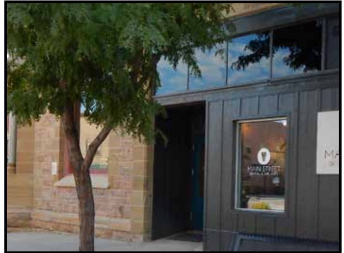
330 Main Street, Reynolds- McGee Building. Original display windows and kickplate had been previously removed in a manner that would presently not comply with the HPDG.
