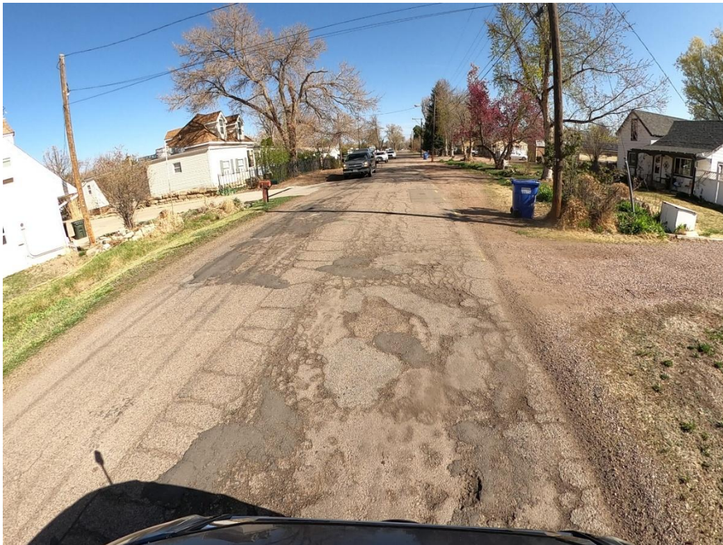
Figure 7: PCI Range 10 to 25 - Serious S Cottonwood Ave between Fowler Ave and E Main St – Actual PCI 17.1
