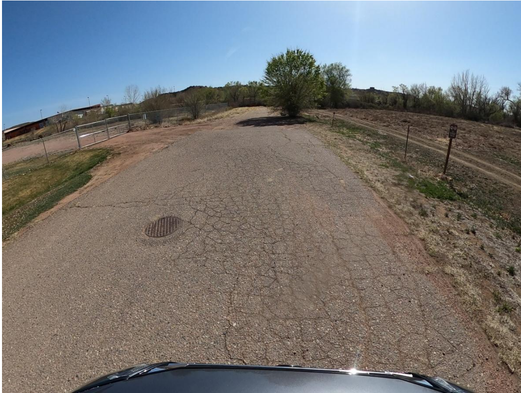
Figure 6: PCI Range 25 to 40 – Very Poor Independence Rd between Justice Center Rd and East End – PCI = 32.0
