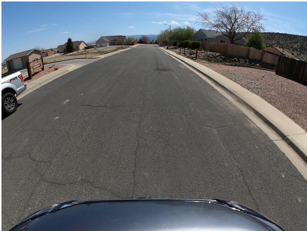
Figure 3: PCI Range 70 to 85 – Satisfactory N 5 th St between High St and Skyline Loop – PCI = 76.9
