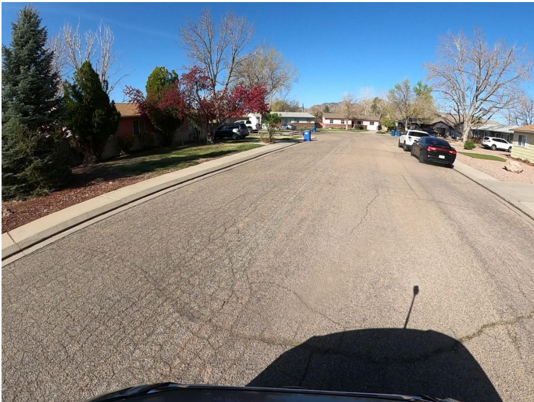
Figure 5: PCI Range 40 to 55 – Poor
