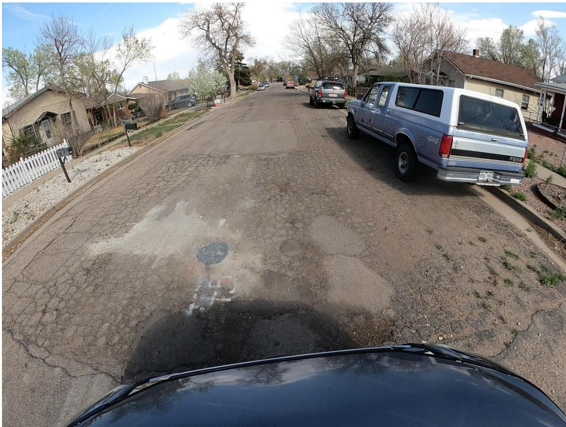
Figure 8: PCI Range 0 to 10 – Failed Allison Ave between N 9 th St and N 10 th St – PCI 6.1
