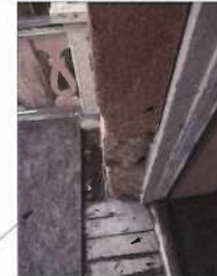
7 Reference Photo -Upper Front Porch A3.1 NTS
