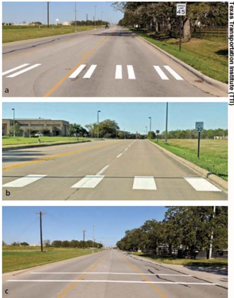
Researchers at Texas A&M University studied the visibility of three types of crosswalk patterns installed on campus: (a) bar pairs, (b) continental markings, and (c) transverse markings.
